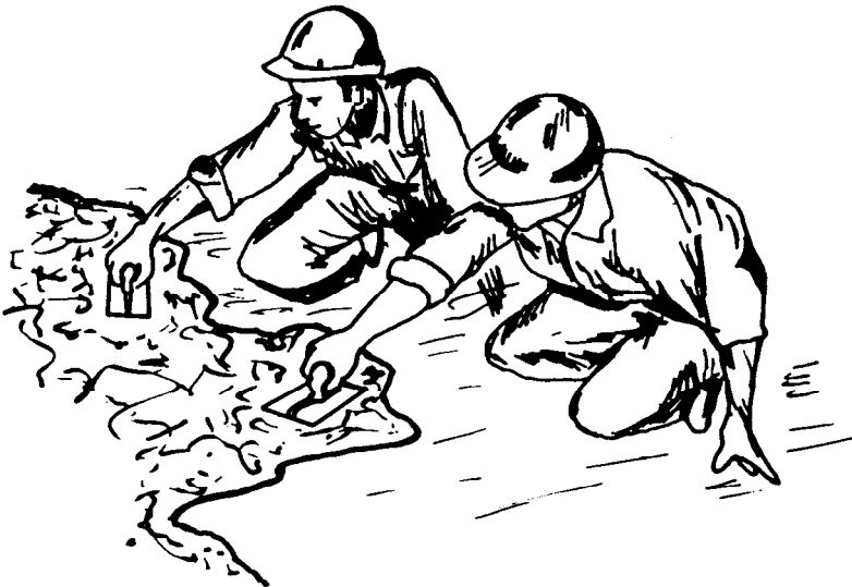
Figure 9-5: Applying a floor coating by hand.
